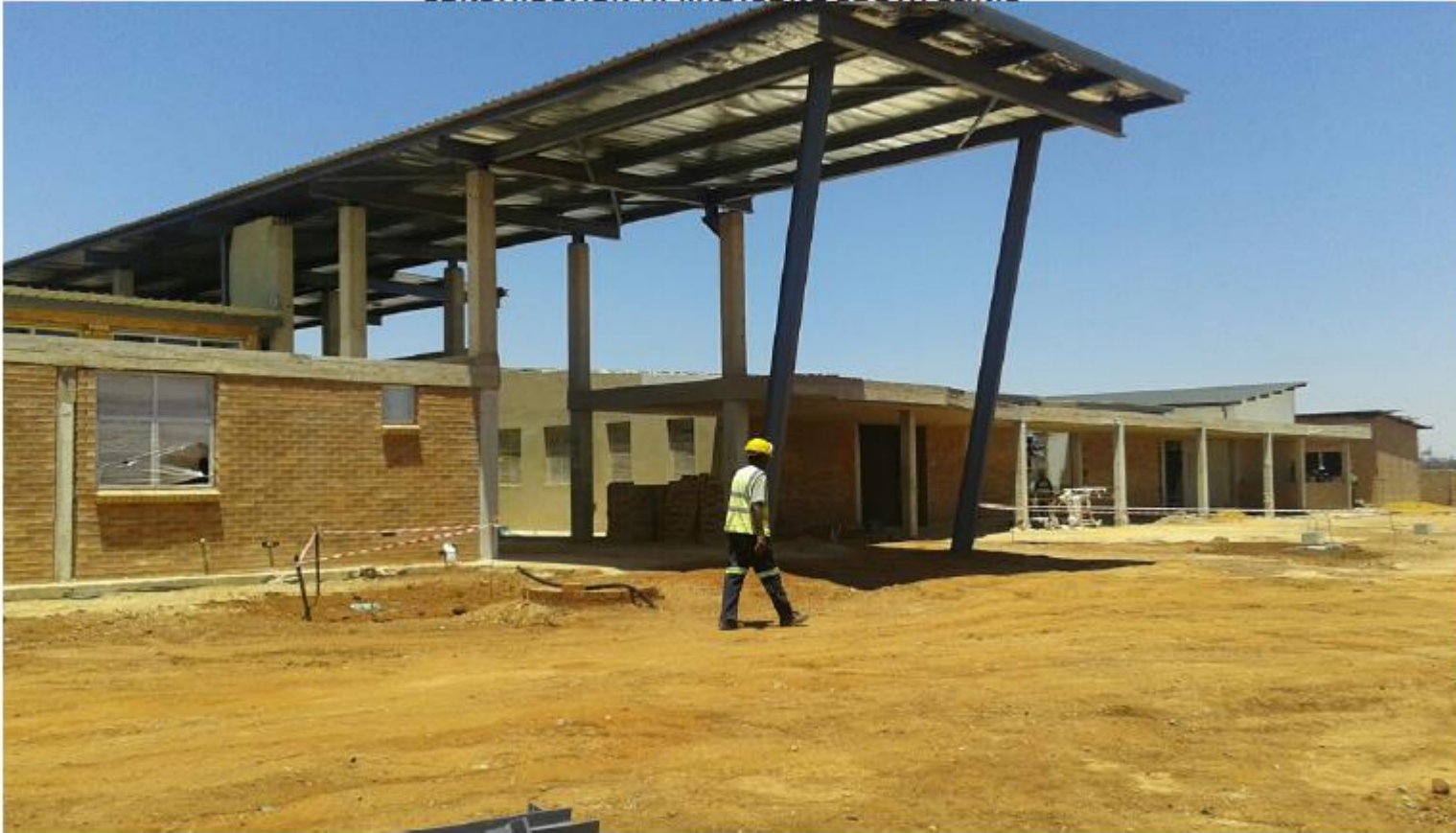
CONSTRUCTION AT KHUTSONG SOUTH CLINIC
